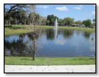
The pond also provided an attractive water feature for a passive park constructed on the premises. With proper maintenance, this wet detention system will provide much needed relief from nutrient loading in the Halifax River and will provide a closer step for South Daytona to achieve TMDL requirements of its surface waters.
