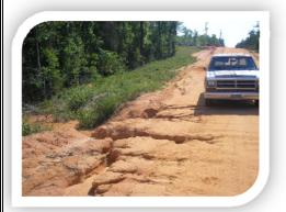
This picture shows the erosion caused by stormwater overtopping the unpaved road. Sediment is washed into the stream.
