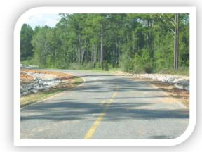
The picture to the right shows the completed section of Trout Toad, fully stabilized. The 6% slopes in the parallel swales are rep-rapped to prevent washout.
