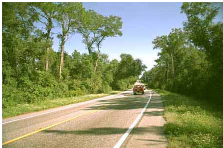
Pensacola Scenic Bluffs Highway Credit: Florida Department of Transportation
