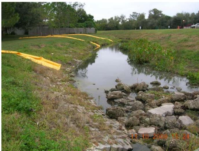
These barriers will not prevent downstream sedimentation with this installation... Even if placed in the stream, turbidity curtains cannot stop downstream sediment transport if there is a significant flow velocity.
