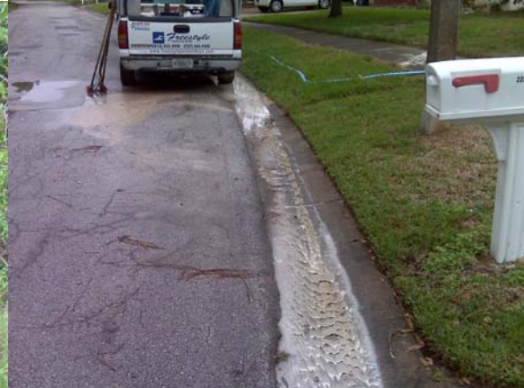
Gary Halstead - PC Public Works / Pool marcite in curb gutter
