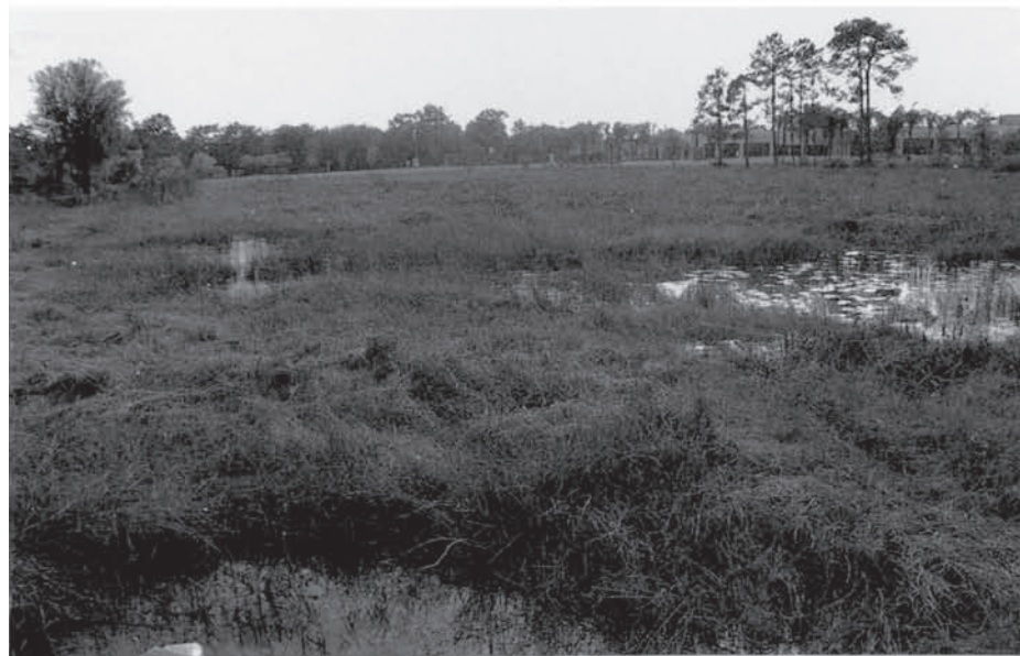
Wetland Treatment System
